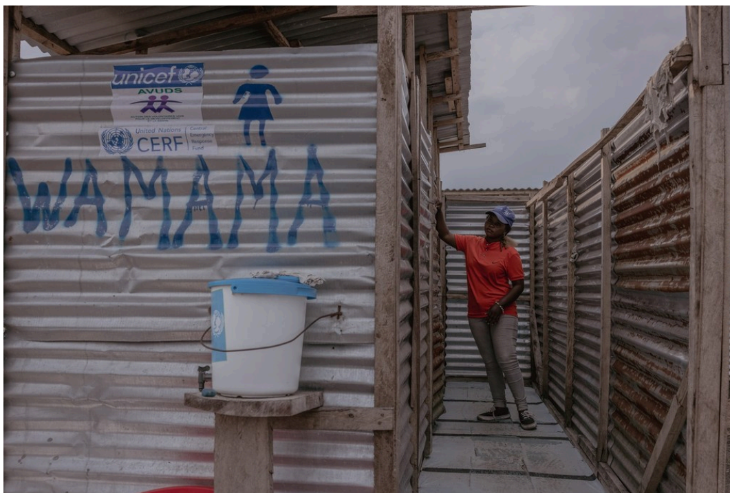
© UNICEF/Ndebo | Toilets installed by UNICEF and its partners in the Bulengo camp, west of the city of Goma, Democratic Republic of Congo.
