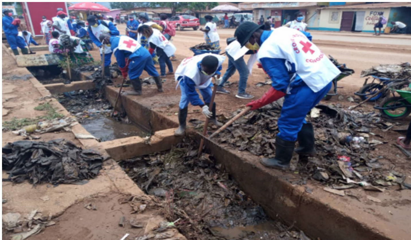
Clearing a drainage channel during a sanitation campaign in Dolisie
