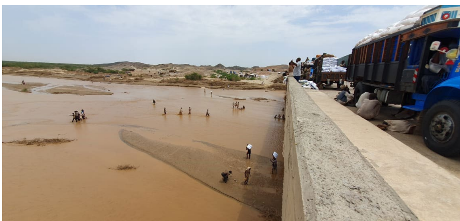
People forced to offload humanitarian supplies due to the collapse of the Khor Baraka bridge in Tawkar locality, Red Sea State (Photo: Lokuju Peter/OCHA)
