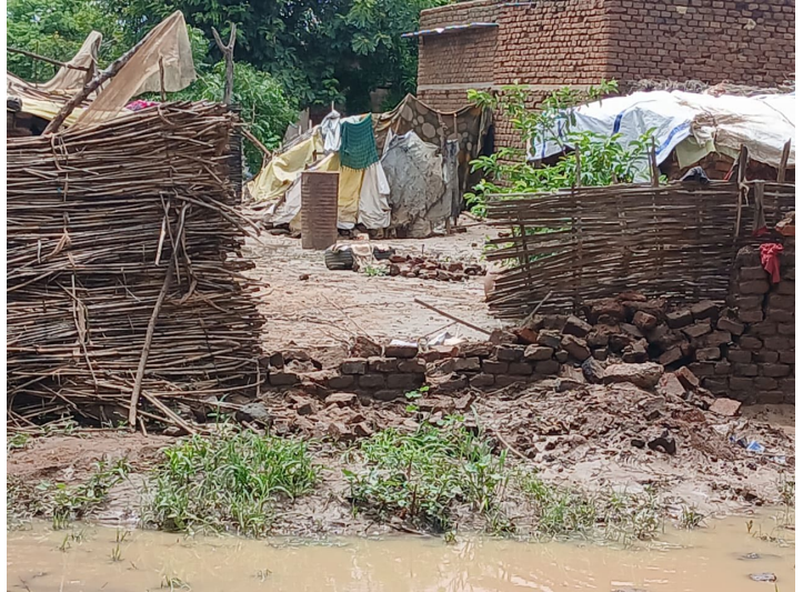
A home damaged by heavy rains in South Darfur Photo: IOM Sudan
